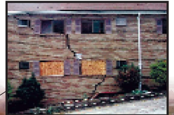
The illustration depicts the typical surface effects of mine subsidence. It is important to note that mine subsidence can occur as a result of mining at any depth. As a general rule, the total surface area affected by subsidence increases as the depth of mining increases. This means a structure can be damaged by subsidence even if is located directly above a pillar or solid block of coal.
